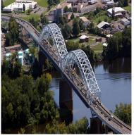
The **Arrigoni Bridge**, also known locally as the **Portland Bridge** is a steel through arch bridge carrying Route 66 and Route 17 across the Connecticut River, connecting Middletown, Connecticut, to Portland, Connecticut. When it opened in 1938, the 1,200 feet (370 m) bridge was the most expensive bridge ever built in Connecticut, at a cost of \$3.5 million. Its two distinctive 600 feet
